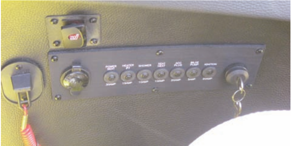
Figure 2-13. Circuit Breaker Panels
